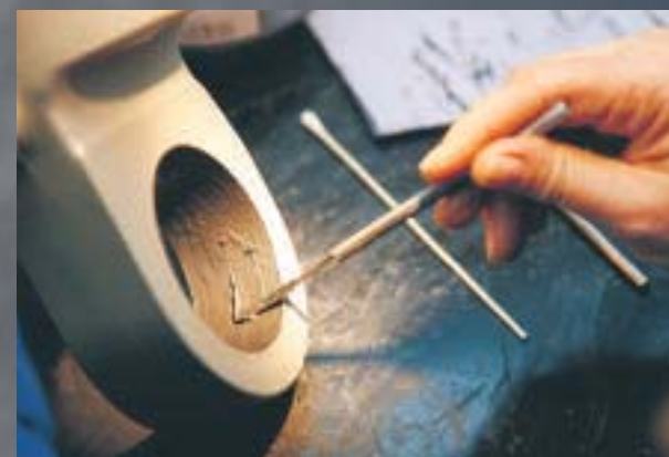
The Interfill® material has to be applied carefully – without any air pockets.
